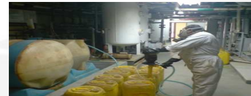
Chlorine dosing for municipal water
