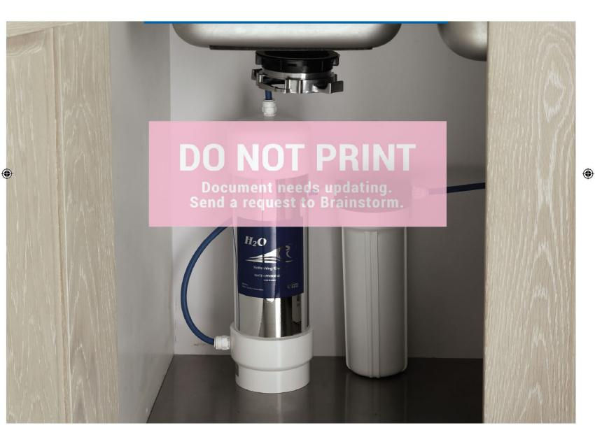
This range of water purifiers caters specifically to the hospitality industry. These purifiers are installed inline to provide your chosen tap, faucet or dispenser with purified water.
