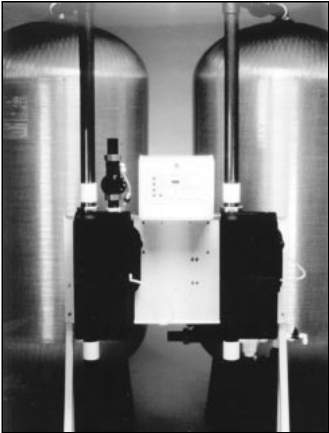
Figure 17 – Two-Bed Deionizer
